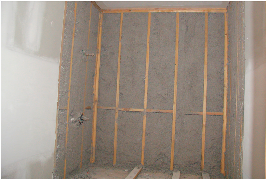
Poor installation of insulation increases the likelihood of condensation inside the basement walls and within the insulation itself. Install insulation behind framing or with furring strips placed against the foundation wall.
